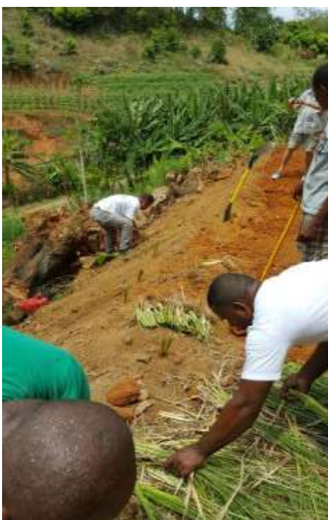
Vetiver grass planted on the riser of the terrace
