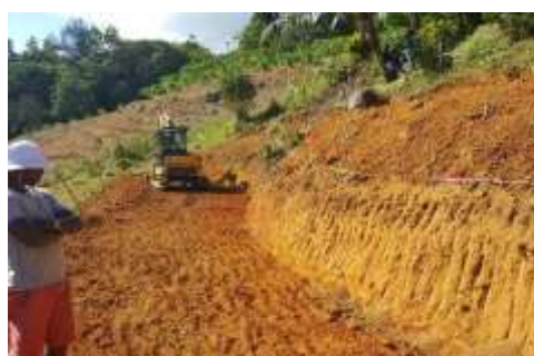
Digger making the terrace on the demarcated contour line
